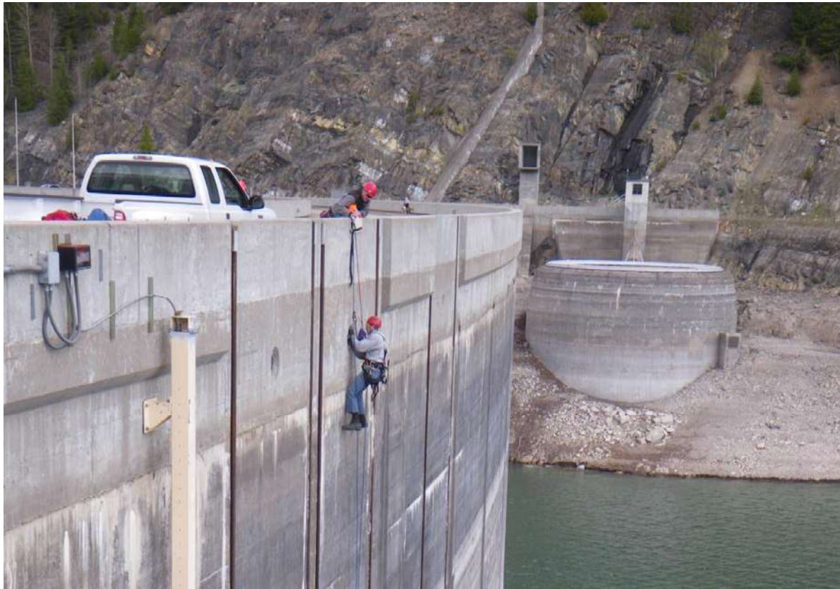
Figure 15. Ropes Team Inspection, Hungry Horse Dam, Hungry Horse Project, Montana.
